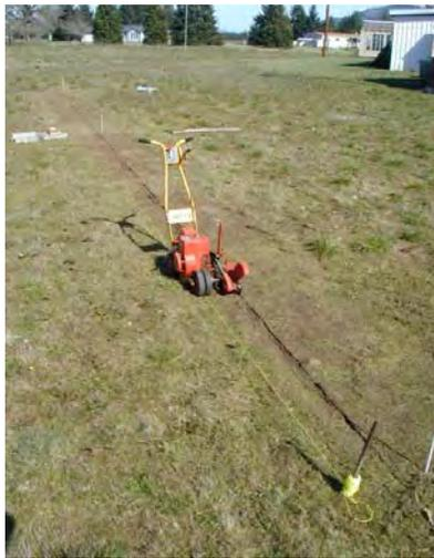
Figure 19 — Cutting a slot in the soil for the 40 foot buried dipole.
